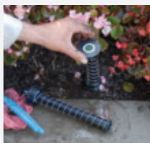
Remove the "guts" of 1806 spray head
